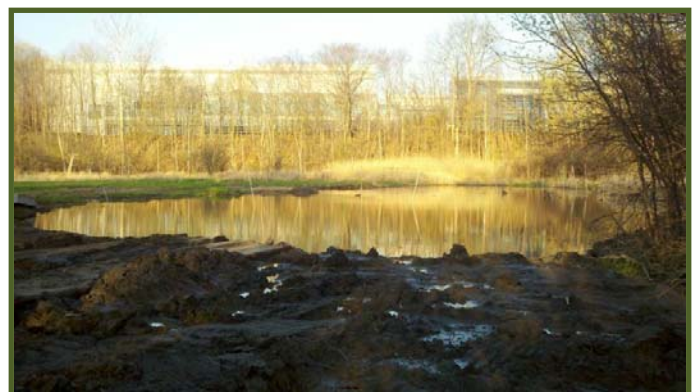
March 29, 2012 – Open water area after excavation completion view from east side of open water, looking west
