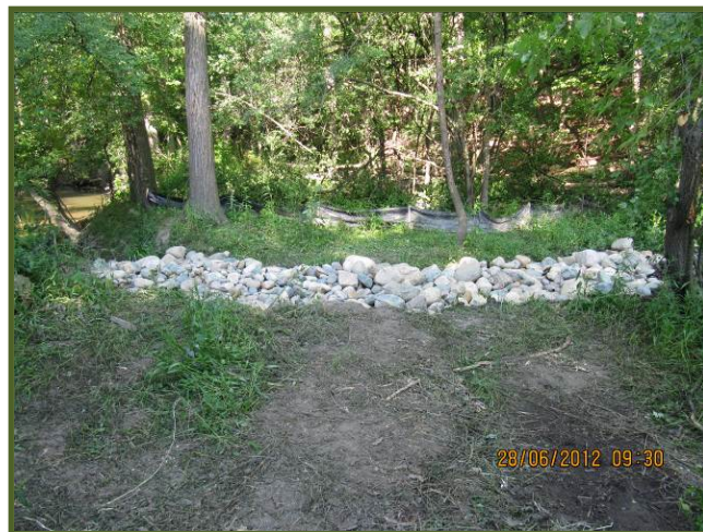
Field stone at west ditch
