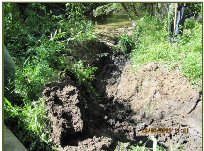
Western south ditch being prepared for plugging
