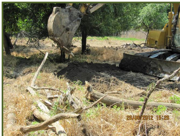
Fill at east ditch
