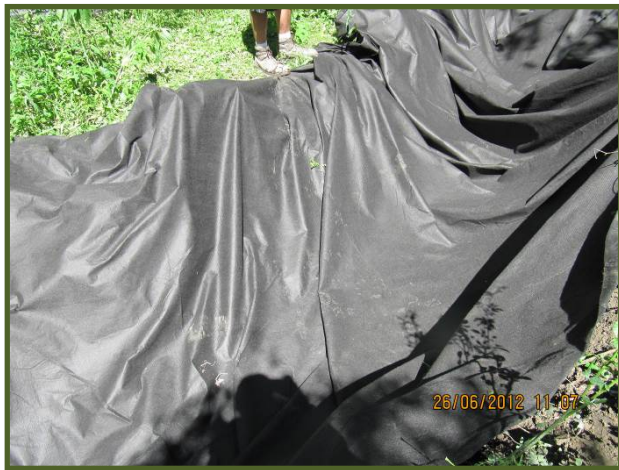
Geotextile fabric lining ditch
