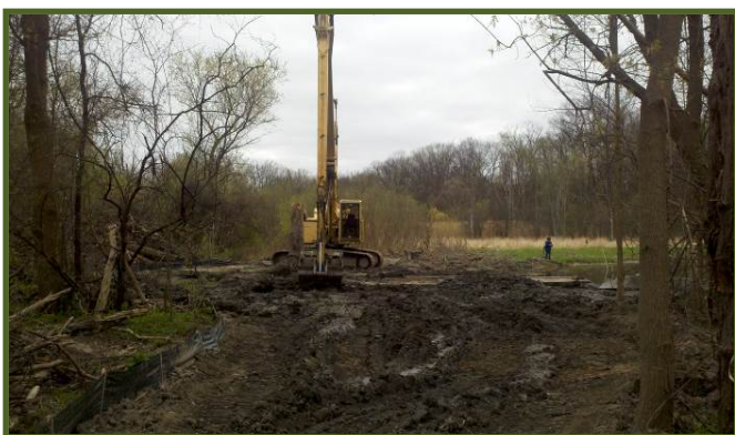
Access route near excavation work area
