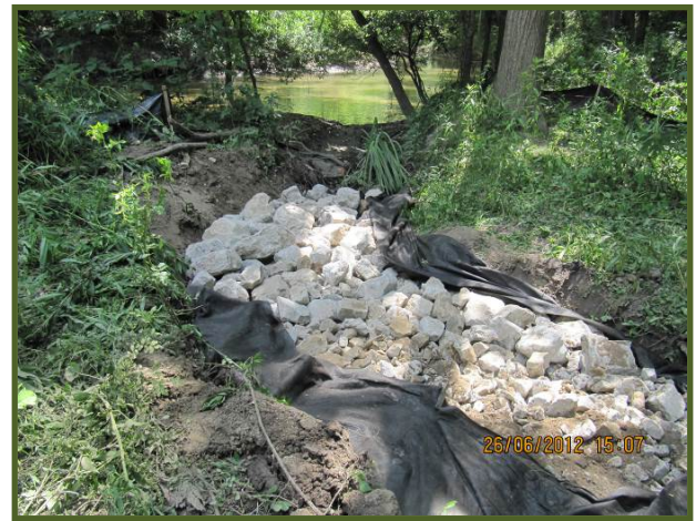
Riprap placed in ditch
