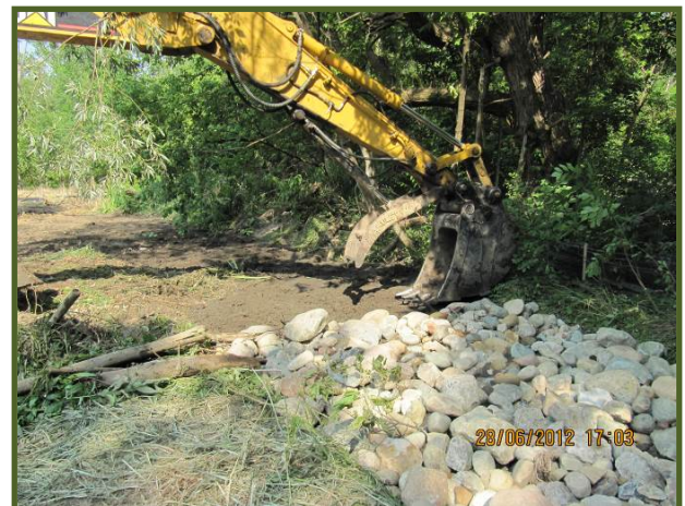
East ditch, fill being smoothed, field stone in place
